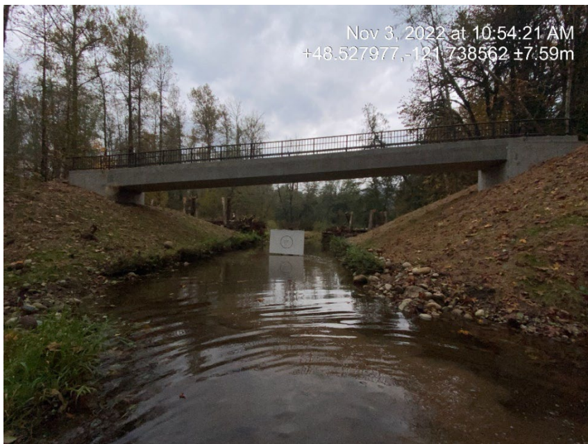
Newly completed bridge at Overnell Slough which replaced a culvert (represented by white square below bridge).
