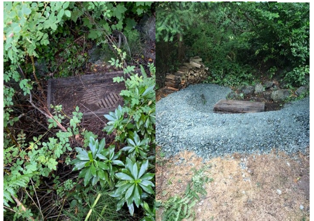
Chiquita Lane catch basin berm improvement (before and after)
