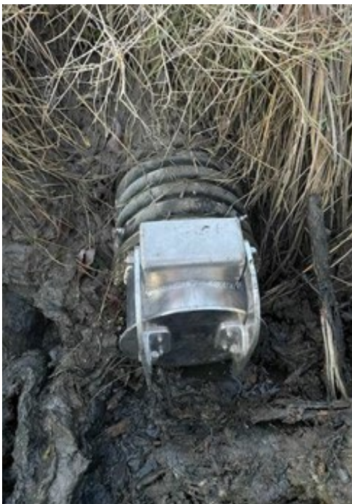
Edison Slough Flapgate Installation
